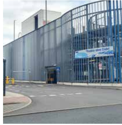
P5 Parkhaus EDEKA Ferdinand-Happ-Straße 61
